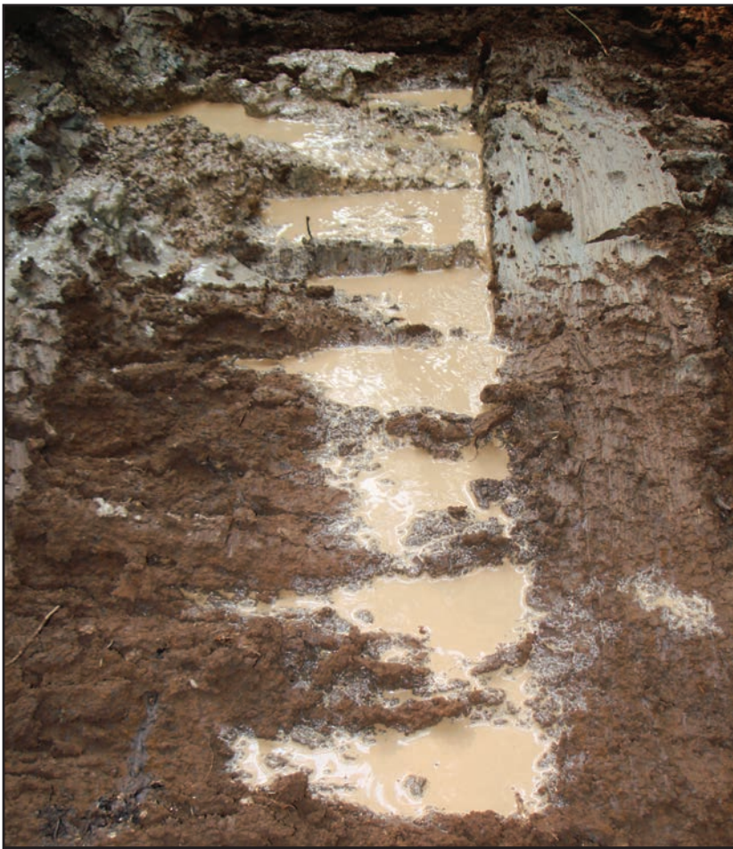
When initial excavation reveals heavy clay soils and water seepage, you may have found the ideal location for a pond.
