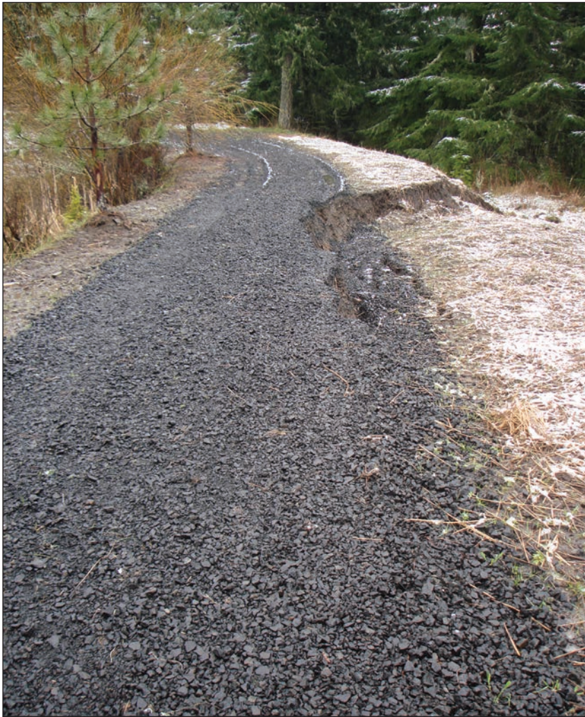
Soil movement caused by ponds can damage poorly placed roads, leading to costly repairs and environmental damage.
