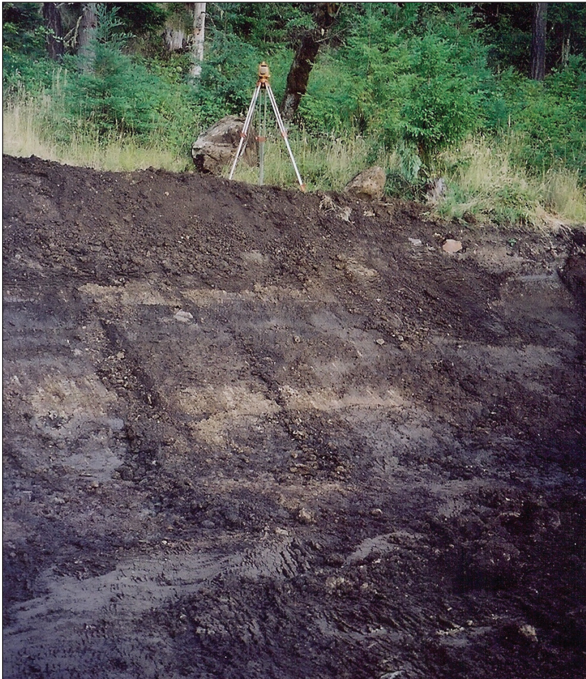
A laser level should be located where it can remain out of the way throughout the construction project.
