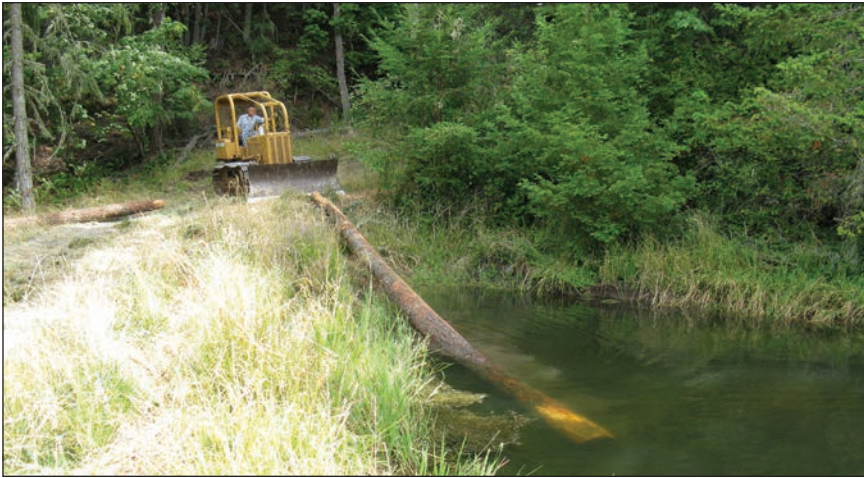
It's much easier to use heavy equipment to put habitat-enhancing logs into the pond.
