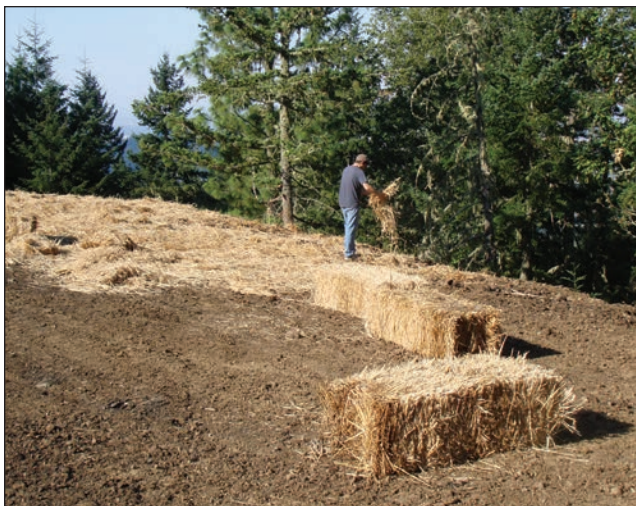
A pond builder spreads out straw along the downslope of the excavation site where the pond will be. Straw makes an excellent weed deterrent and is an environmentally sound way to control both weeds and erosion. The straw will also attract a variety of wildlife.
