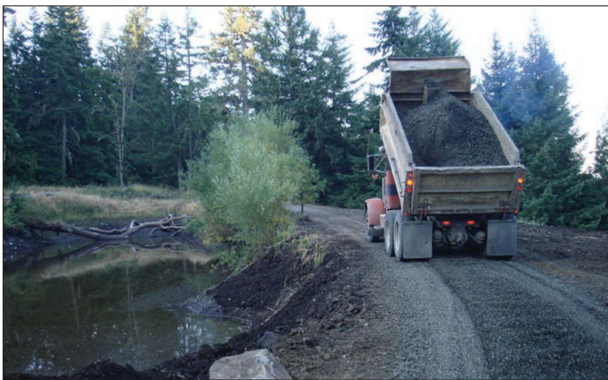
A dump truck can be used to remove soil from a pond site and then used to deliver and spread rock along the road.
