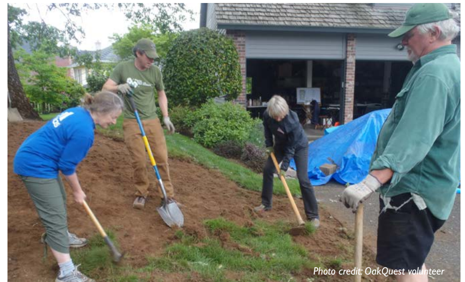
Stripping sod by hand
